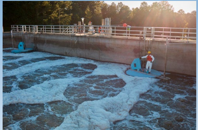
Maintenance Supervisor Jamie Veley at the Rose Creek Wastewater Plant in Woodstock, Georgia, USA.
